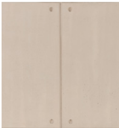
Concrete Panel Encofrado
